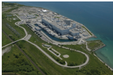
Figure 1 CANDU reactor facility
