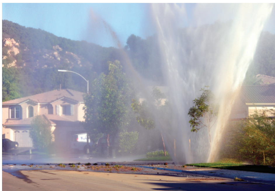
Figure 8 When pipes freeze and burst, it can be a big mess, both above ground on road surfaces and below ground in water and sewer systems.
