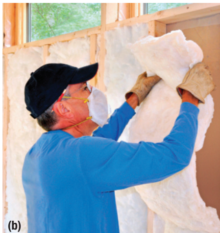
Figure 8 Thermal insulators include (a) fur, (b) fibreglass, and (c) foam insulation. All of these materials trap air and help to prevent the transfer of thermal energy from an object to the surroundings.
