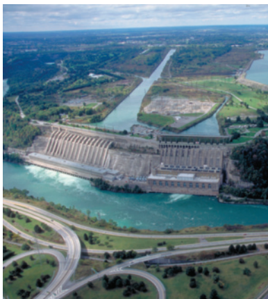
Figure 1 This hydroelectric power plant is transforming the kinetic energy of the falling water into electrical energy.
