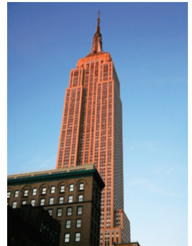
Figure 3 The Empire State Building in New York City was built using massive concrete walls to reduce vibrations.
