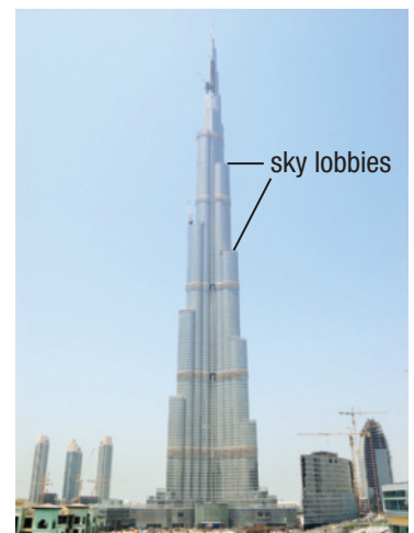
Figure 4 At 828 m, the Burj Khalifa, in Dubai, is the tallest structure ever built. Notice the sky lobbies in this structure.
