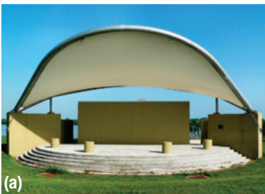
Figure 3 (a) A concave wall reflects sound to a single focal point. (b) A convex surface reflects sound so that the sound waves are dispersed. (c) Flat surfaces reflect sound evenly.
